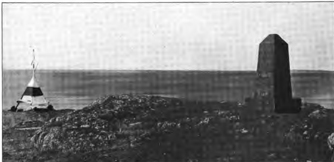
PILE POINT REFERENCE MARK.
